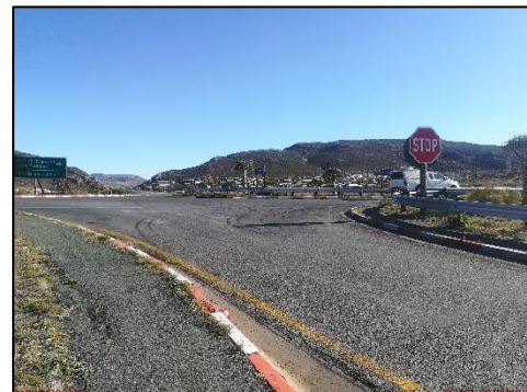
Pic 5 - Tight right-turn at N7 off-ramp intersection with R355 (near Springbok)
