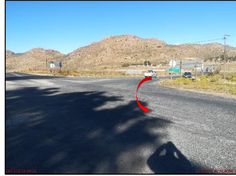
Pic 6b - Tight left-turn at R355 intersection with the N14 (viewed from N14)
