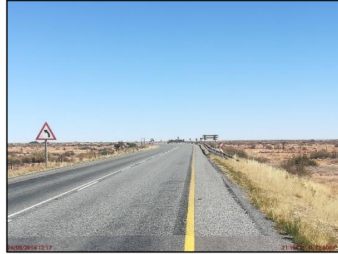
Pic 17 - Viewing west from M759 along N14
