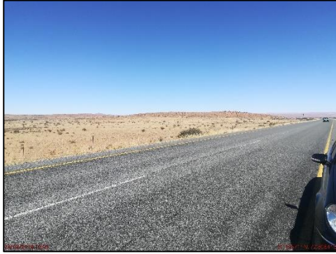
Pic 10 - Westernmost end of site (viewing west towards Pofadder)
