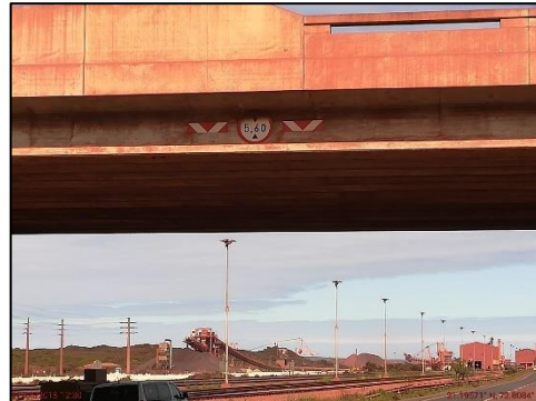
Pic 2 - 5.60 m height restriction bridge on roadway leading from Saldanha Port
