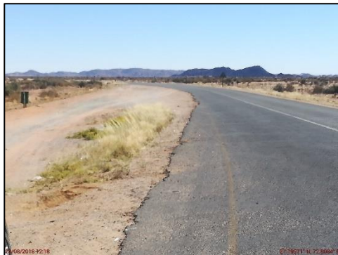
Pic 18 - MR759 viewed from its intersection with the N14
