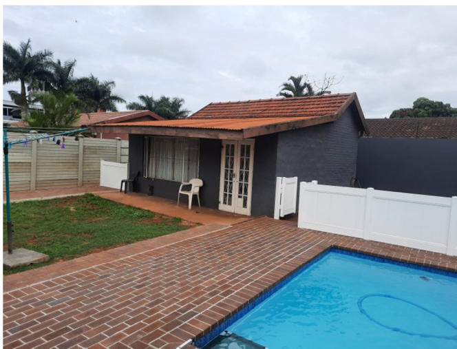
View across pool towards existing Outbuilding – proposed Pool/ Entertainment Room to be situated where the white fence is located – to be built after approval.
