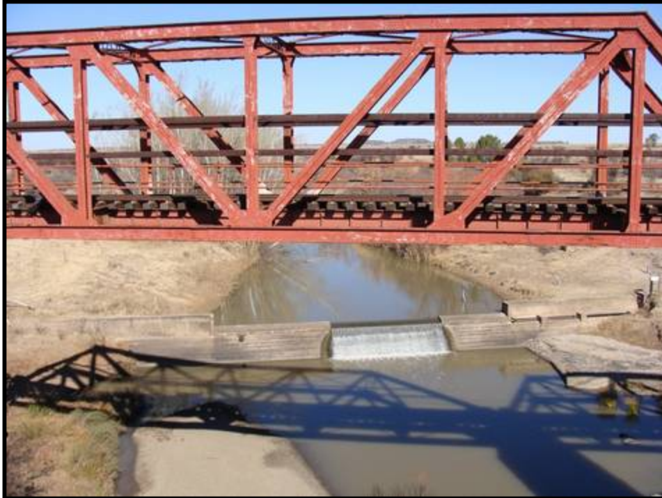
Photograph 3.3: Modder River and rail bridge from the N8
