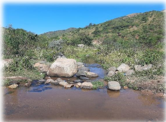
Photo 19: Downstream photo of a reach of SE-Transitional River-468 at the location of a causeway road crossing.
