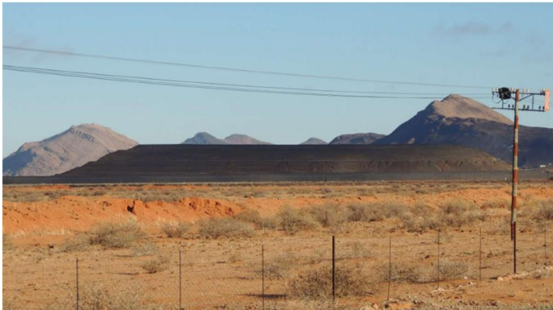
Figure 22: Photograph from the access road to Aggeneys Town of the existing Black Mountain Tailings Storage Facility.
