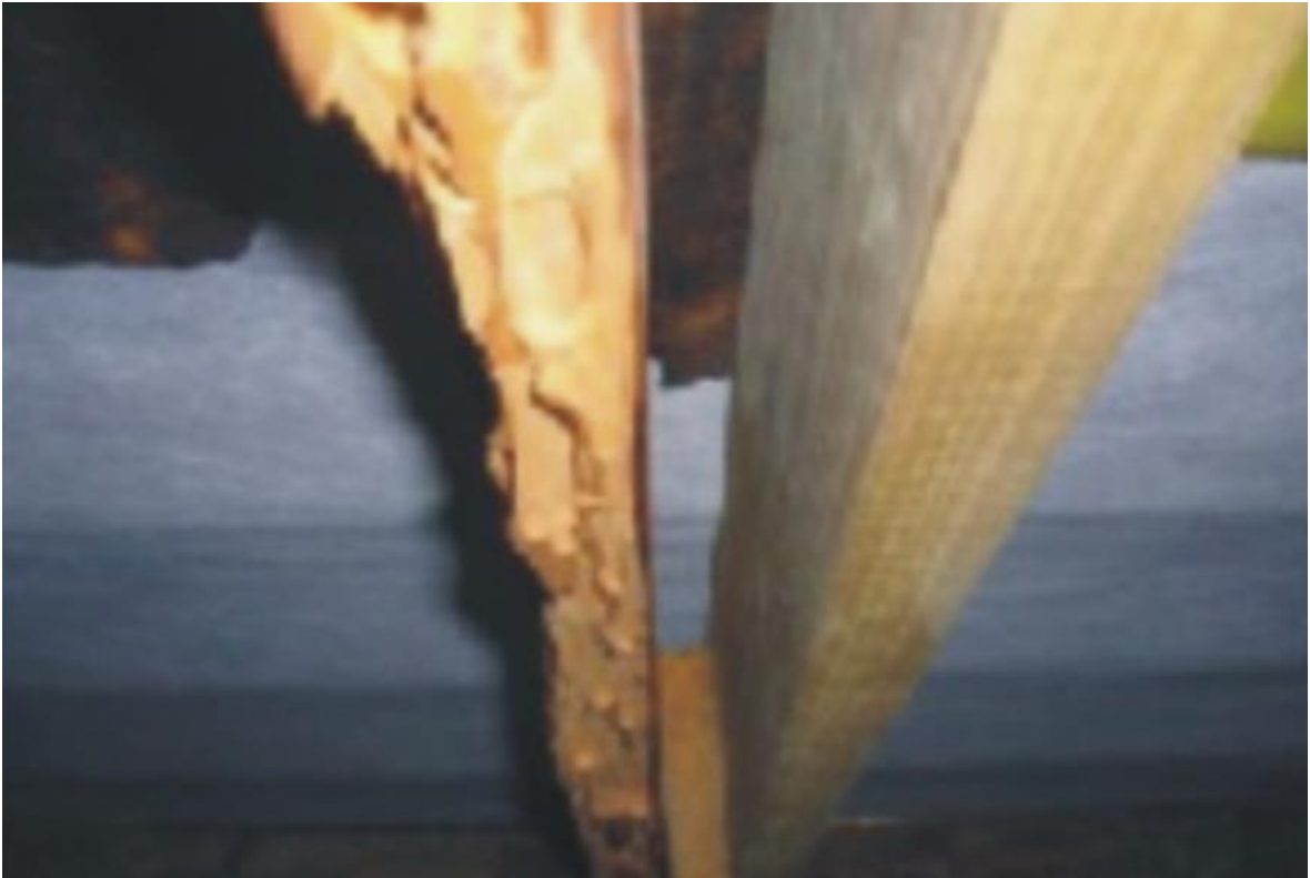
Image 9: View of the damaged roof trusses.
