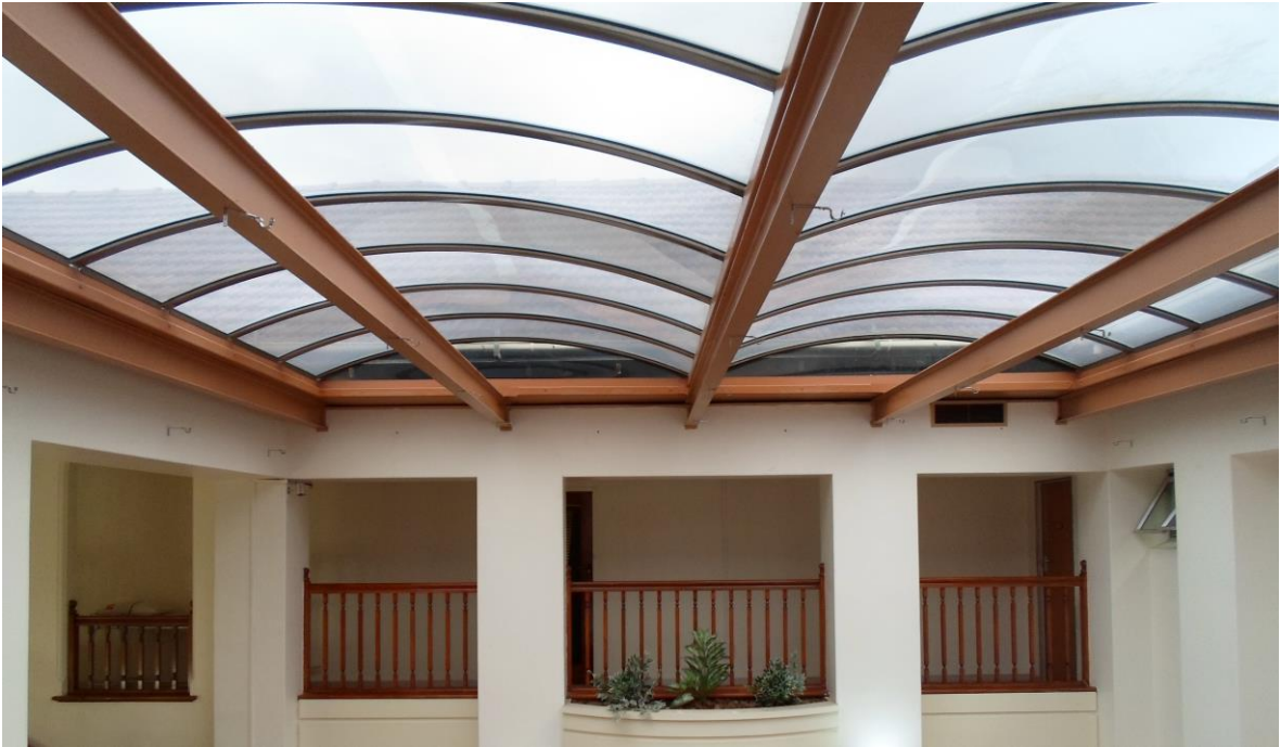
Image 7: Skylight over the foyer of the St Augustine's Medical Centre 2.
