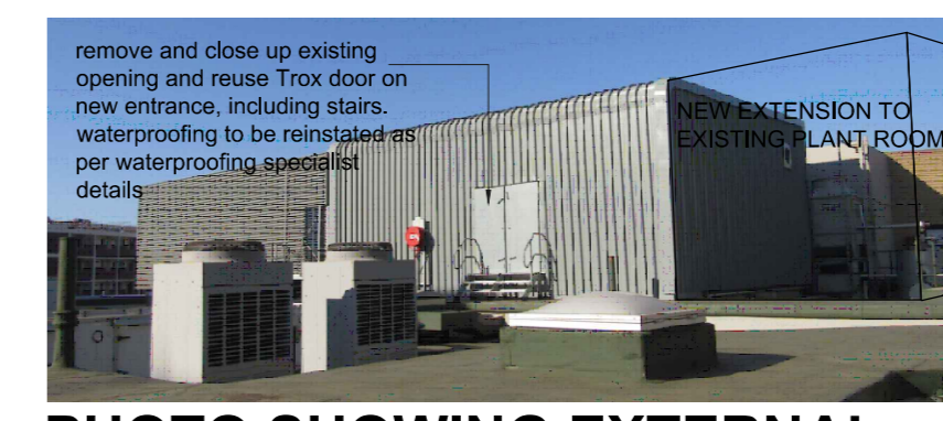
PHOTO SHOWING EXTERNAL OF EXISTING PLANT ROOM
