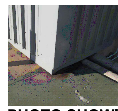
PHOTO SHOWING FOOTING OF EXISTING PLANT ROOM
