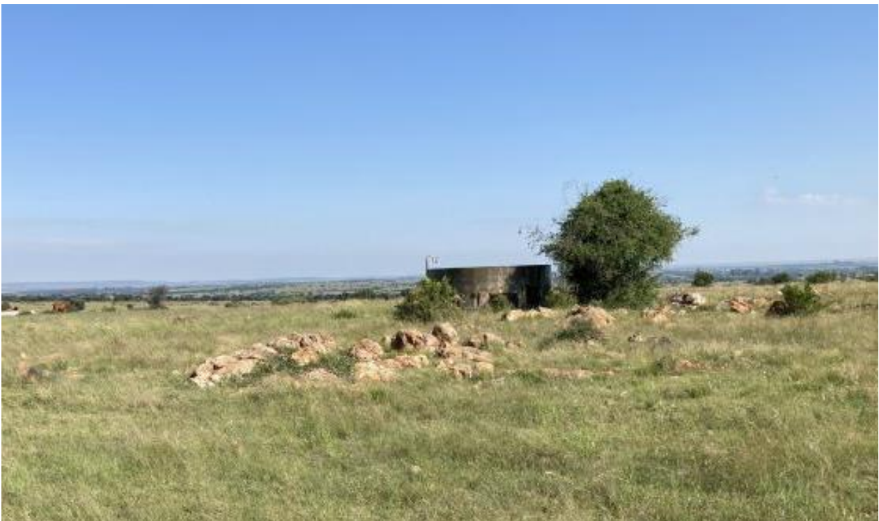
Figure 7: Cement water reservoir in the assessment area.
