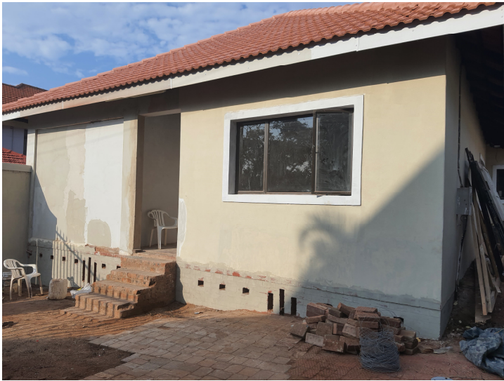
NE ELEVATION FROM NORTH CORNER
