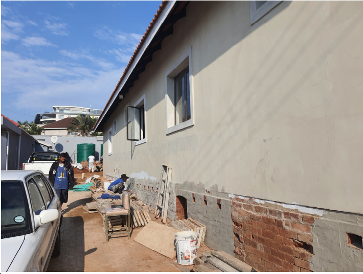
SE ELEVATION FROM THE NE CORNER
