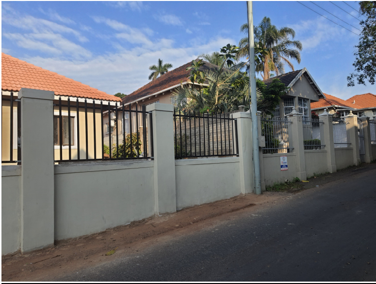
PART NE BOUNDARY WALL INDICATING RIGHT NEIGHBOUR AT 15 PALM GROVE
