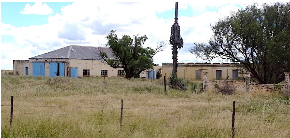
Figure 3: Louwsvilla farmstead to the south of the proposed Kudu Solar PV facilities is derelict
