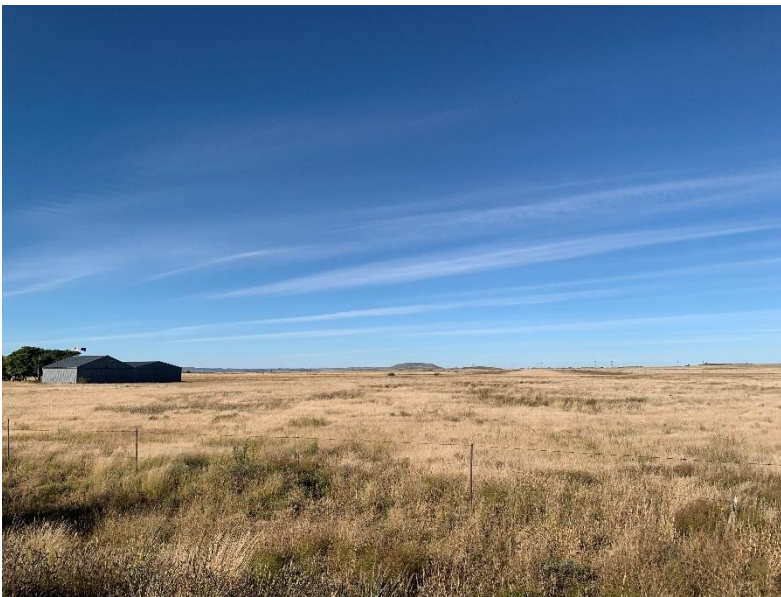
Photo 5: A view of the De Aar airport runway and the airport infrastructure in the lefthand side of the photograph. The runway is very difficult to recognize as it is overgrown with vegetation.
