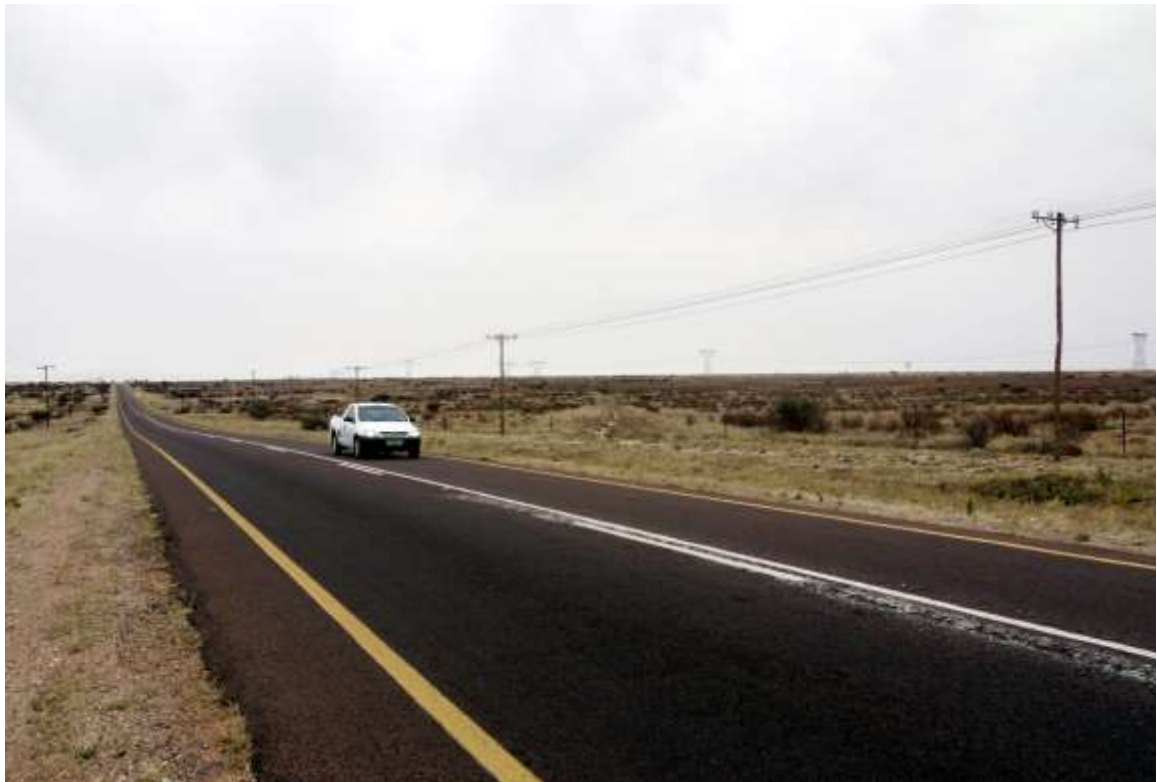
Plate 21, View from VP3 on the N14 approximately 2.5km to the south of the Upington MTS.
