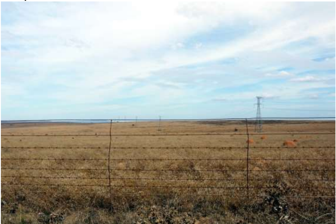
Plate 17 - A view along the line of an existing similar overhead power line with steel lattice towers
