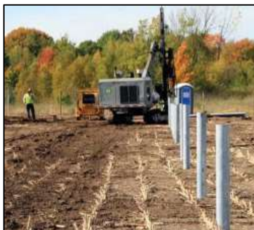
Figure 5: Driven/ Rammed Steel Pile
