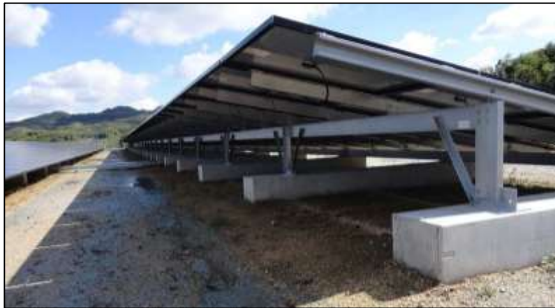
Figure 3: Cast Concrete Foundation
