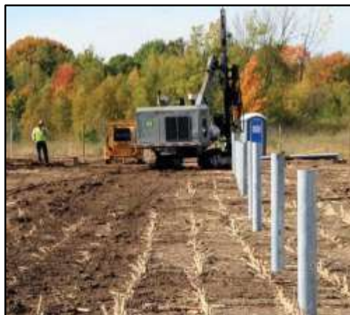
Figure 4: Driven/ Rammed Steel Pile
