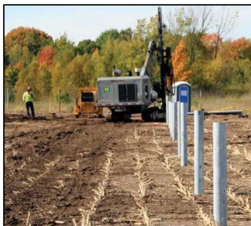
Figure 4: Driven/ Rammed Steel Pile
