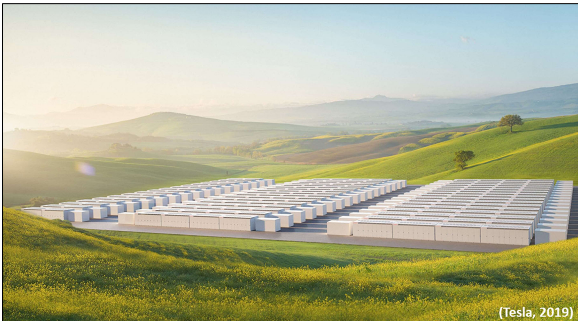
Figure 1: Tesla's Megapack Li-ion Battery (Modular System).
