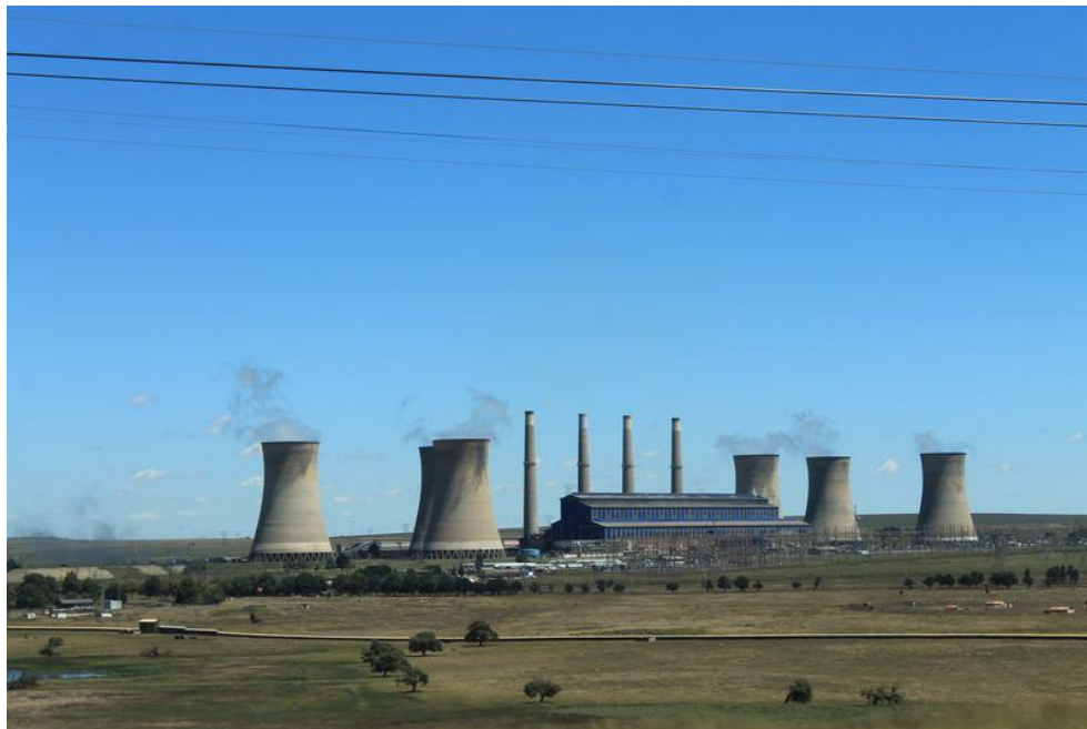
Photograph 3.1: Camden Power Station
