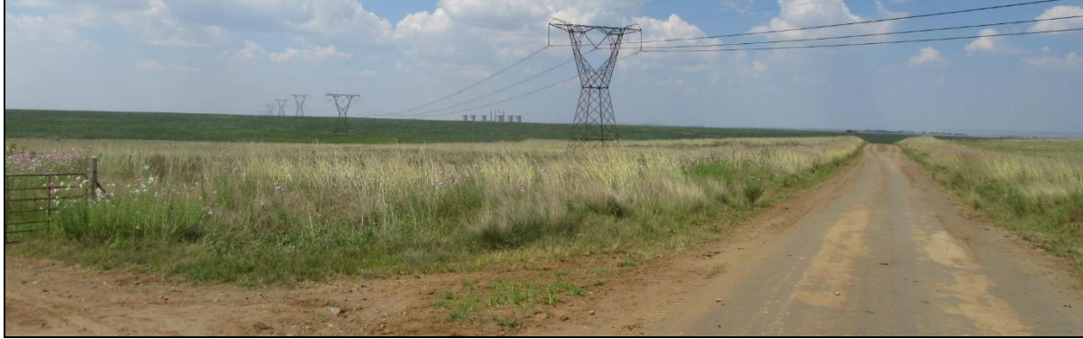
Photograph 3.11: 400 kV line crossing the De Emigratie Road on Uitkomst.
