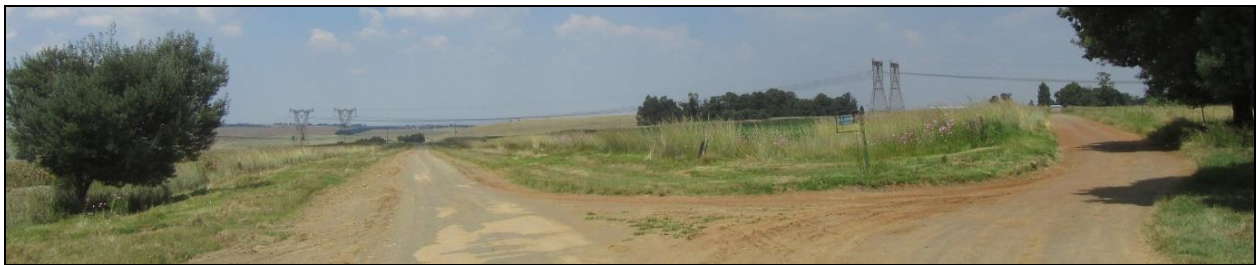
Photograph 3.12: Two 400 kV lines traversing De Emigratie Road
