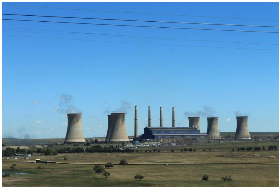
Photograph 3.1: Camden Power Station
