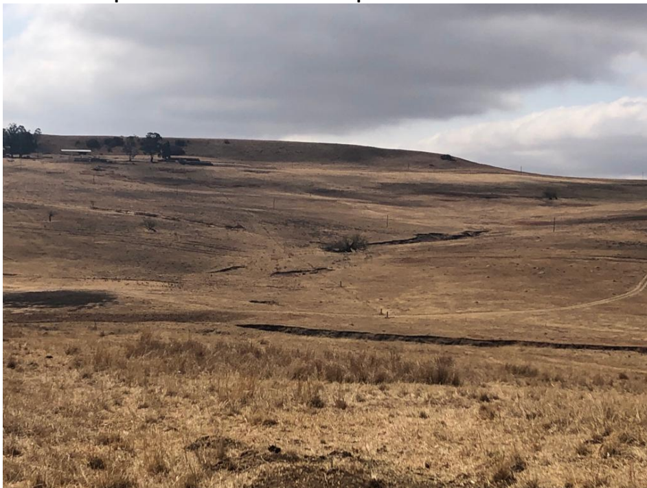
Plate 5: A view of a minor water course, with a view of an earth wall farm dam upstream
