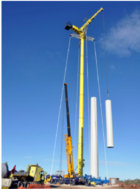
Figure 4-6: Cranes at work
