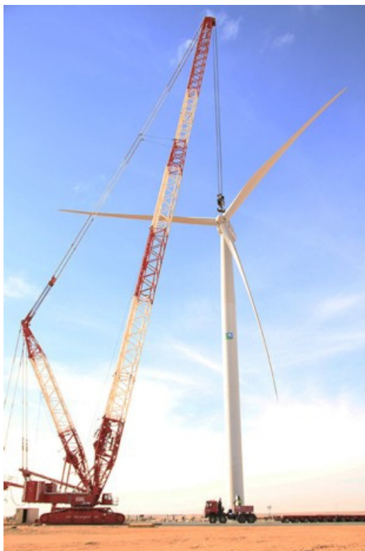
Figure 4-5: Crawler Crane used to assemble turbine (Liebherr, 2017)
