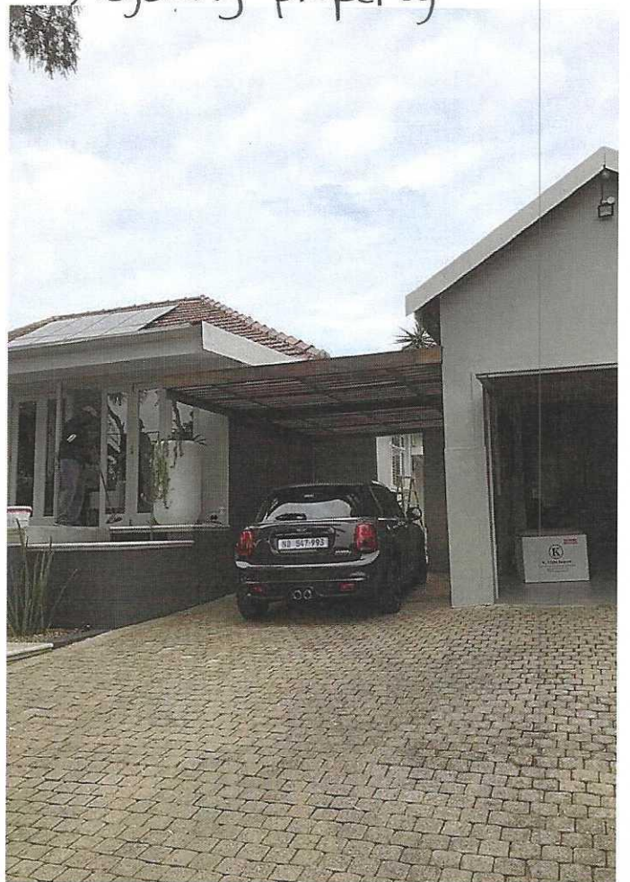
Driveway view - new carport
