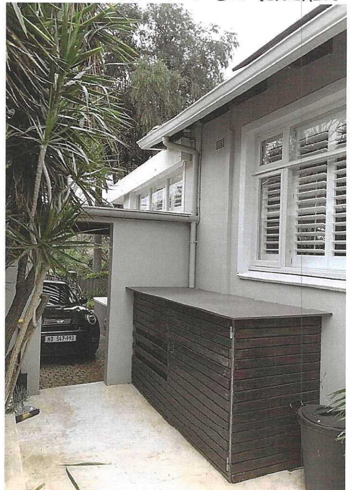
PART WEST ELEVATION & Rear of carport.
