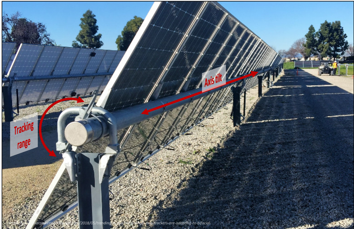
Figure 3.4 – Axis tilt and tracking range
