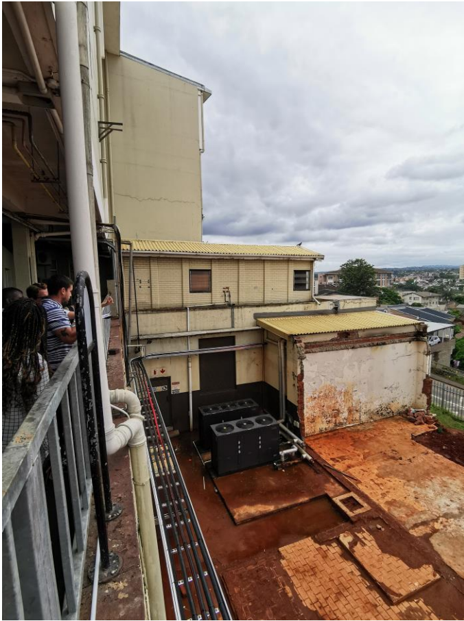
Image 3: View of existing Parklands Hospital.
