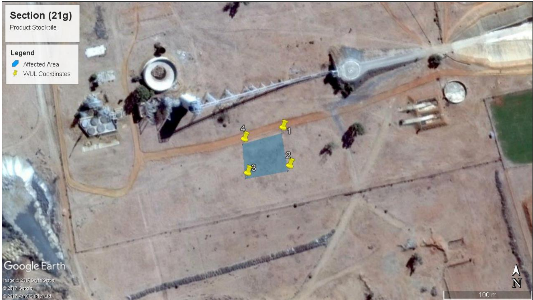
Figure 13: Weltevreden Section product stockpile location (21g)
