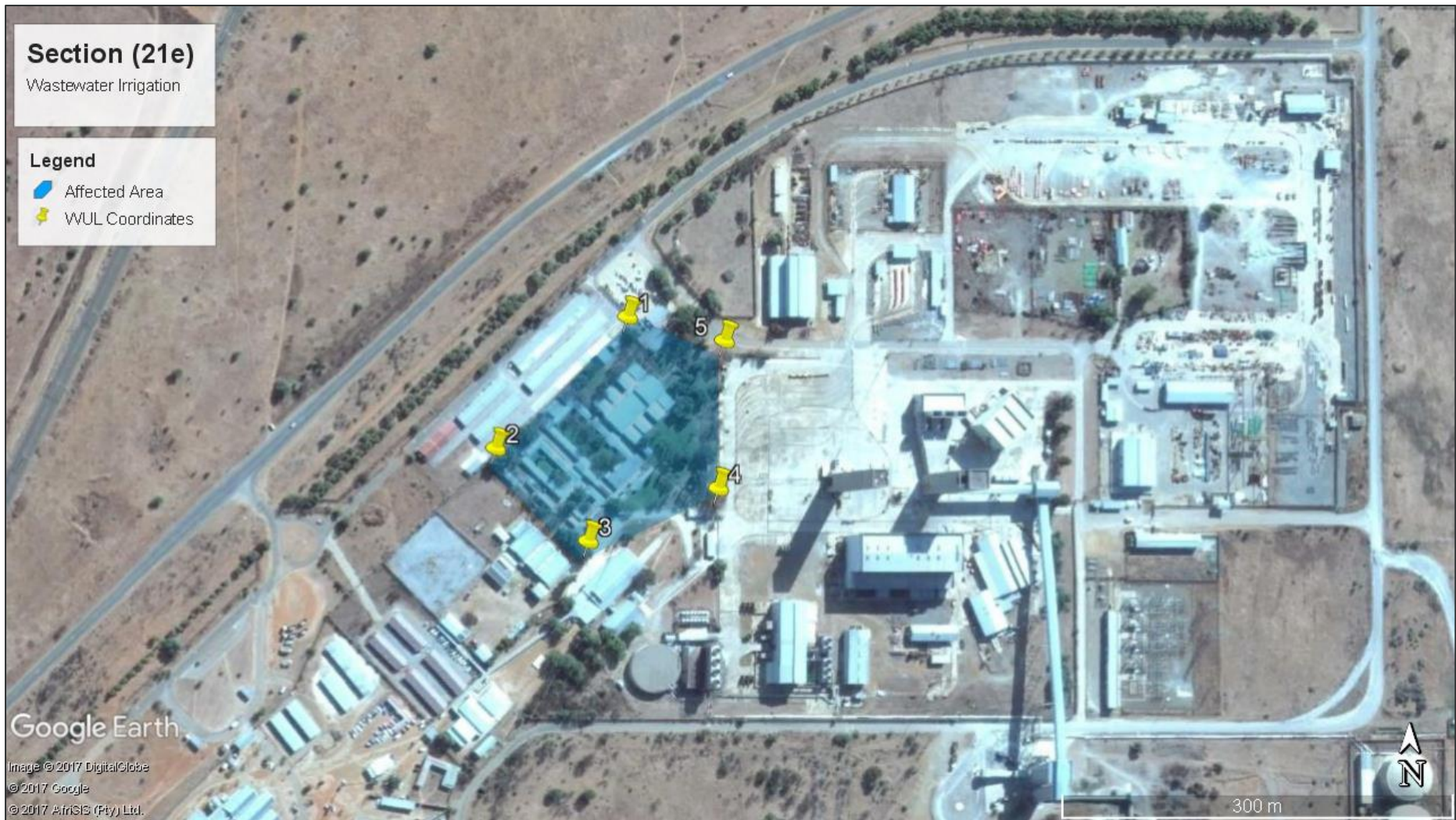
Figure 7: Tau Lekoa Section irrigation of lawns with treated waste from sewage treatment works (21e)
