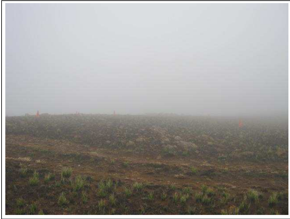
13. General view on site establishment area
