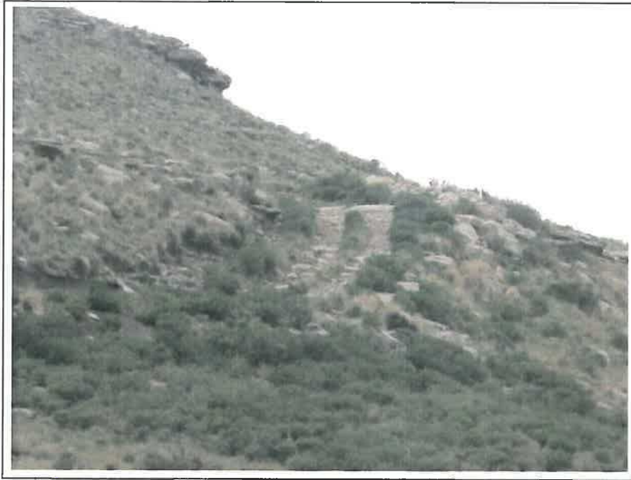
13. General view on existing 2 track access road to site establishment area
