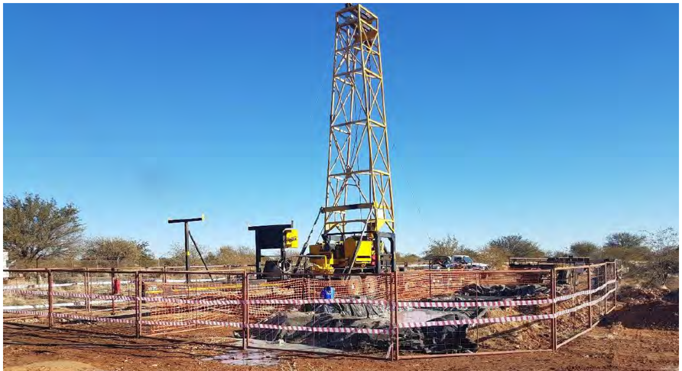
FIGURE 3-1: TYPICAL DIAMOND-CORE DRILLING RIG
