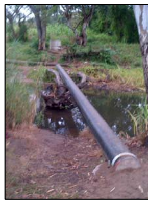
Site Photo 4: Existing 'make-shift' bridge
