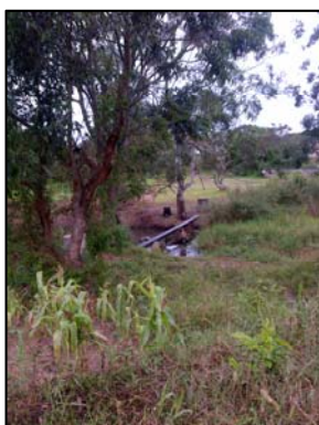
Site Photo 7: Existing pedestrian bridge
