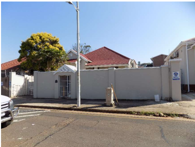
SOUTH EAST ELEVATION - NEIGHBOURING BUILDING ACROSS THE ROAD ON LEFT
