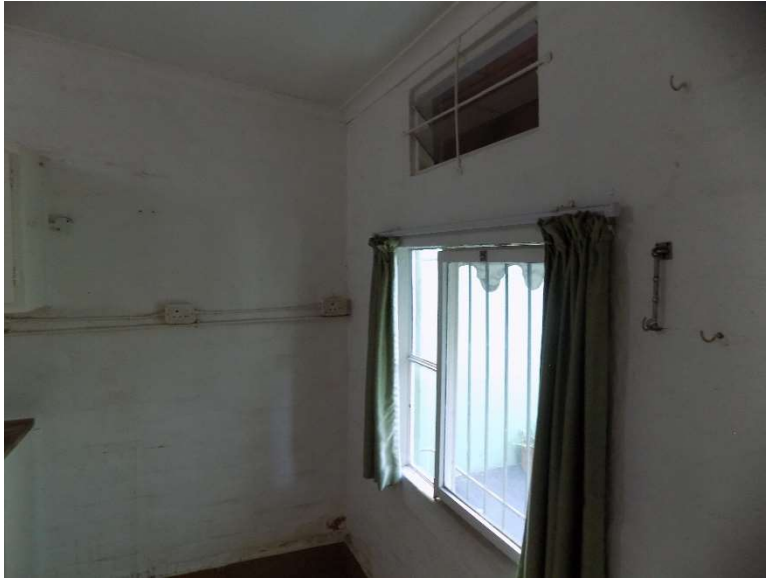
OUTBUILDING- INSIDE OF EXISTING STORE
