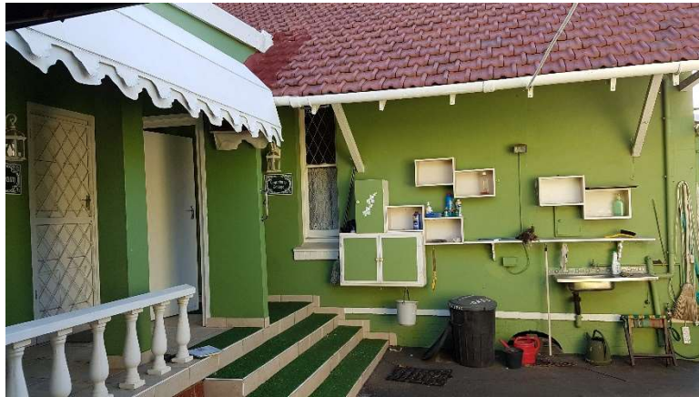
EAST ELEVATION – REAR OF MAIN DWELLING
