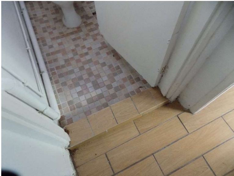
OUTBUILDING- INSIDE OF EXISTING WC
