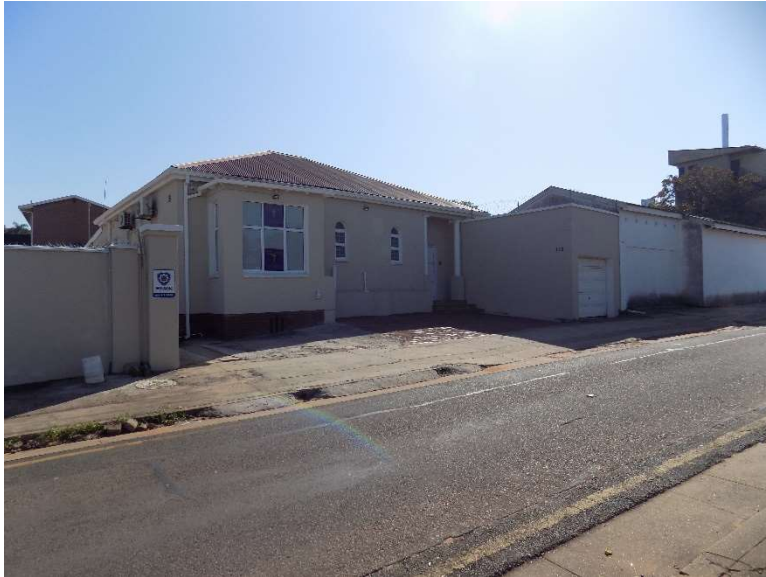
SOUTH EAST ELEVATION – NEIGHBOURING BUILDING ACROSS THE ROAD
