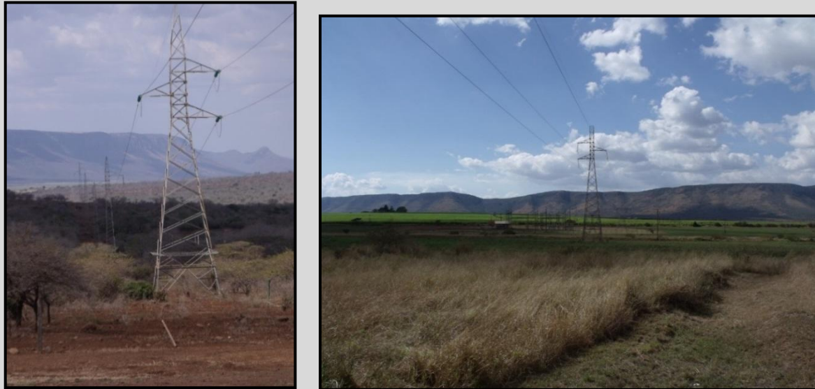
Figure1: Views of the existing power line.
