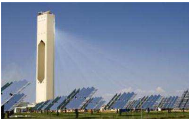
Figure 1-6: CSP in Seville, Andalusia, Spain.
