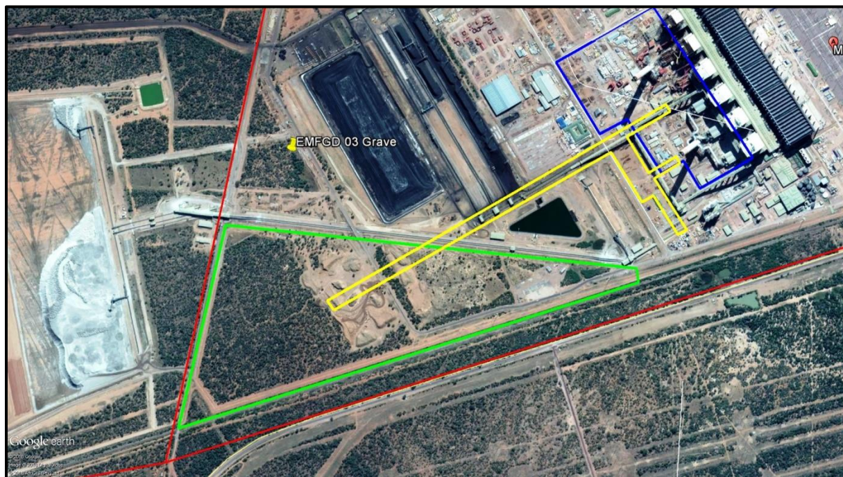
Figure 8-28: Aerial map of the area reflecting the location of a possible grave site between the MPS and ADF
