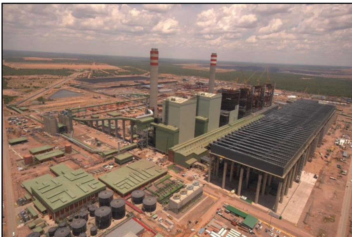
Figure 8-1: Photograph of the construction of the MPS
