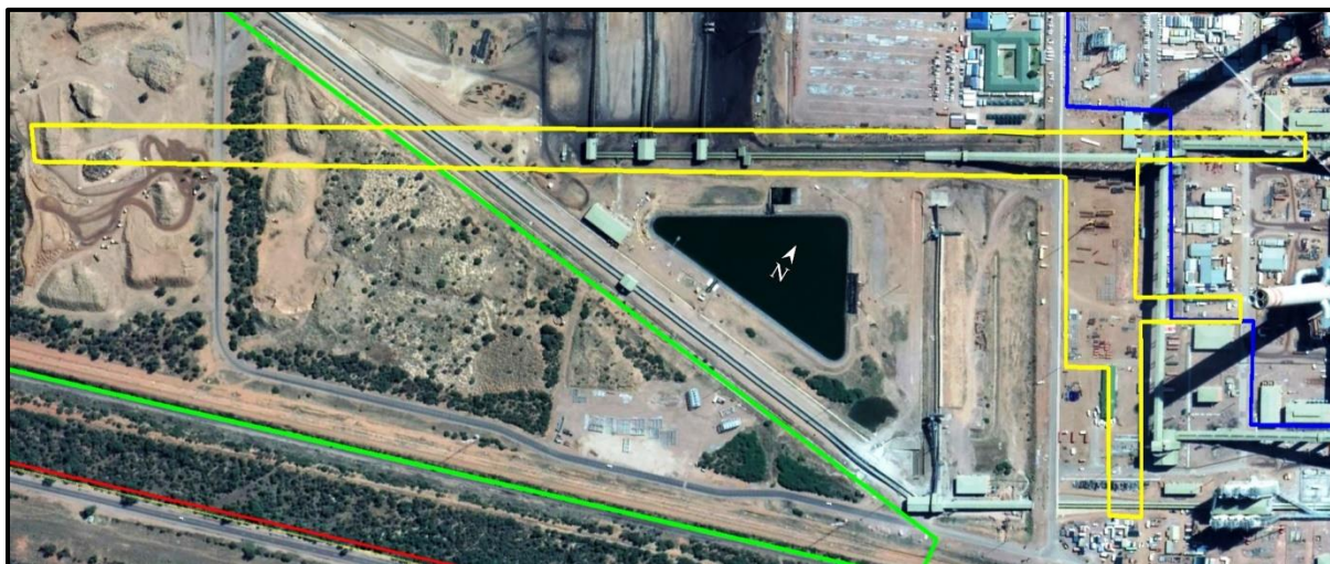
Figure 6-5: Conveyor alignment area linking the rail yard and FGD
