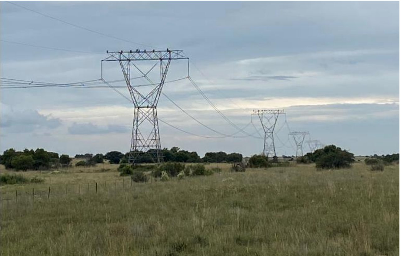
Figure 8: White-backed vultures roosting on the Hermes – Pluto 1 400kV transmission line the assessment area.
