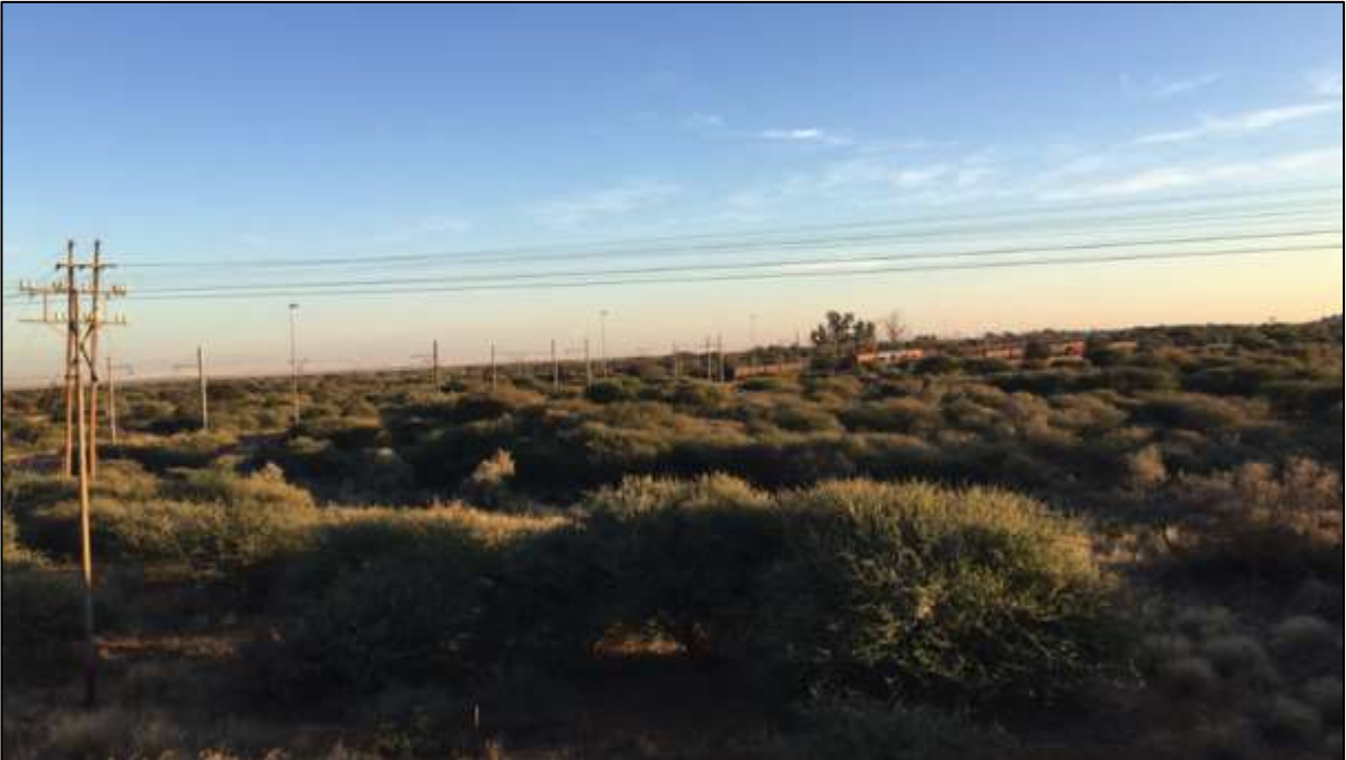
Figure 23: View north from Photo 5 of the existing power line and railway line infrastructure along which the proposed power line would be routed.
