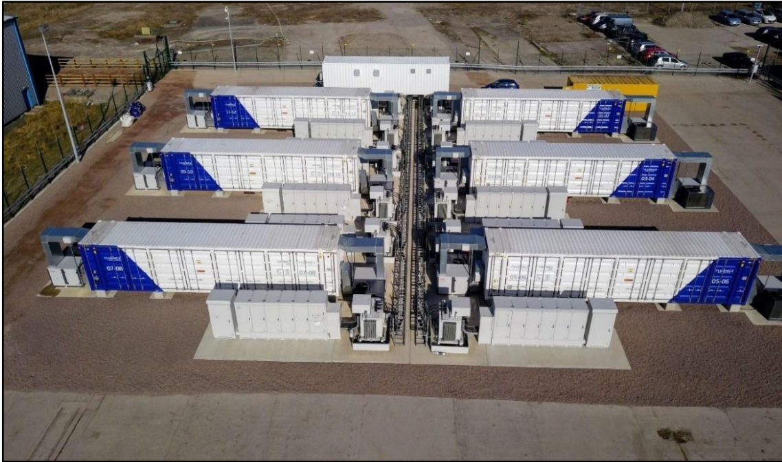
Photograph 1.2: Example of BESS located in storage containers
