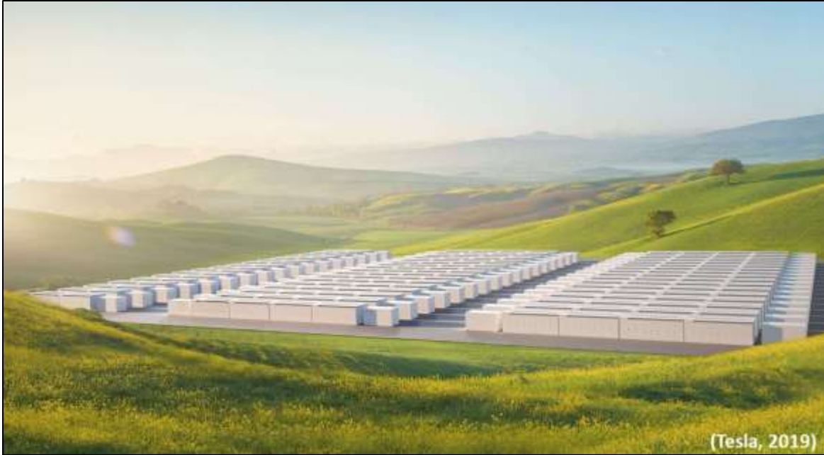
Figure 1: Tesla's Megapack Li-ion Battery (Modular System).
