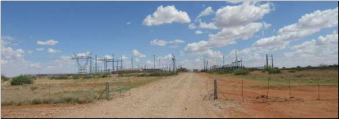
Photograph 3.8: Eskom’s Upington MTN substation seen from the entrance road to the facility off the D3276 gravel road.
