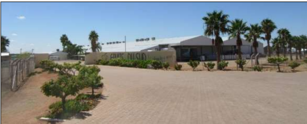
Photograph 3.7: Fruits de Sud’s raisin processing facility near the N14-Kanoneiland Road intersection
