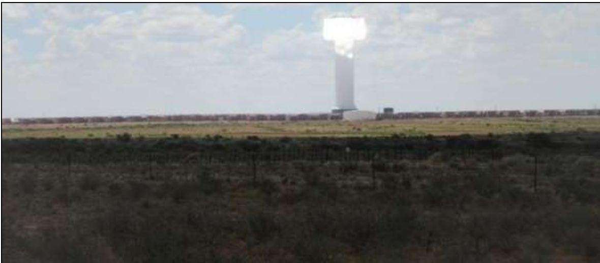
Photograph 3.17: Tower on Khi One SEF, seen from the eastern boundary of Dayson's Klip just to the south of the Daysonsklip 1 SEF site.
