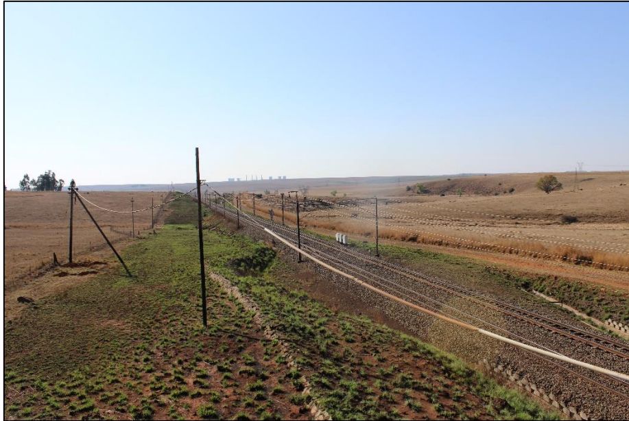
Figure 23: Rail infrastructure and power lines to the south-east of the Camden 1 SEF project area.
