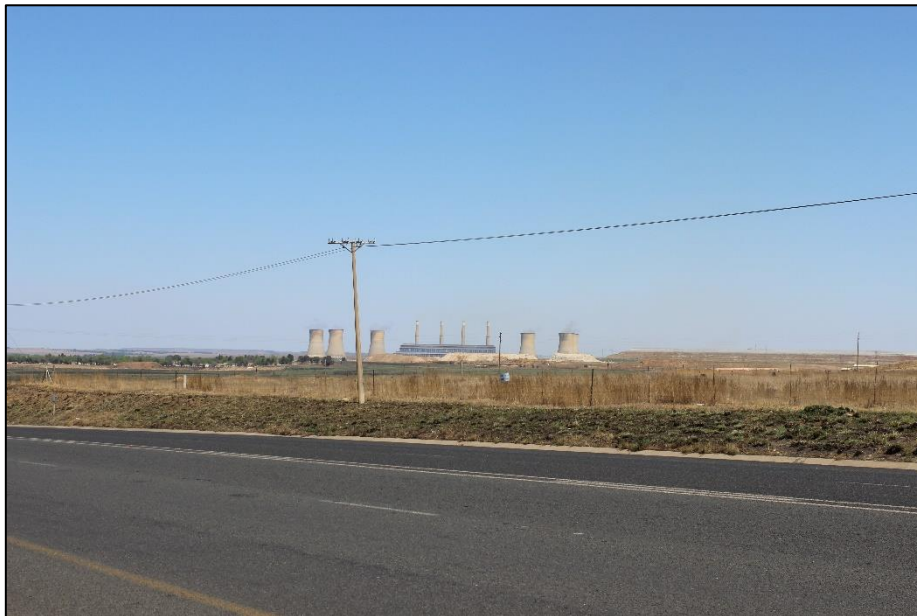
Figure 24: View of Camden Power Station to the west of the N2 national route.
