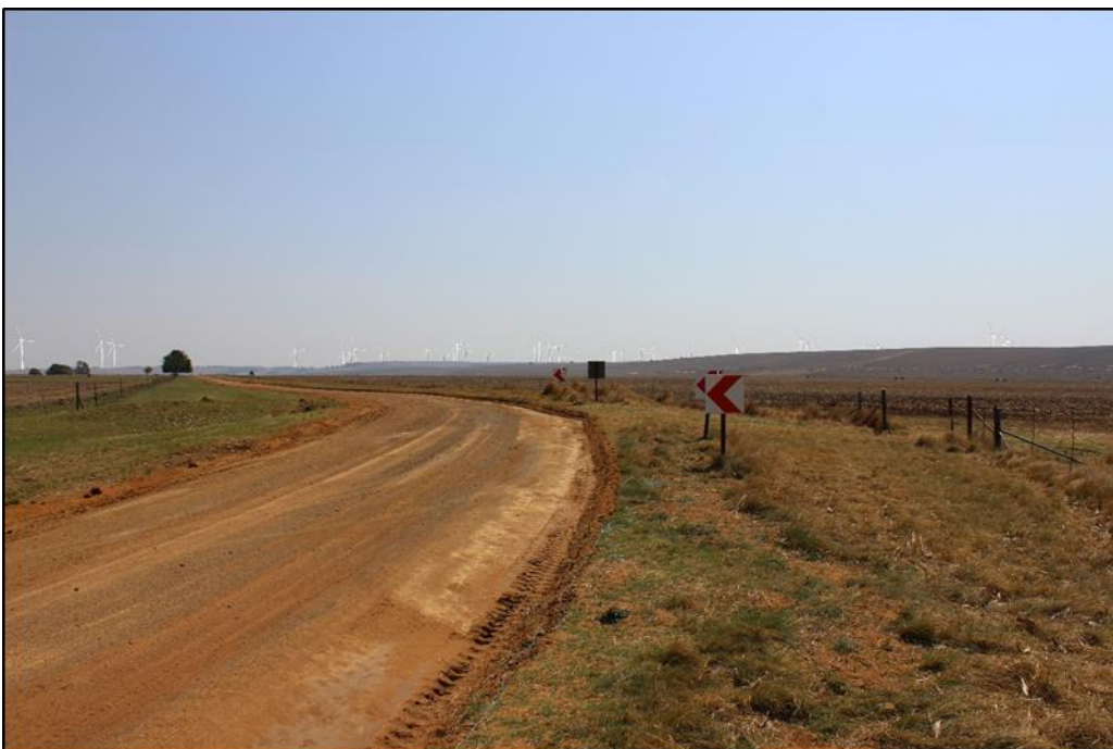
Figure 38: View north from Viewpoint MP3 – Post Construction
