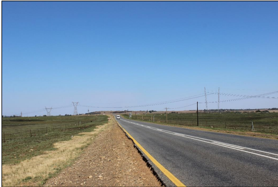
Figure 25: High voltage power lines feeding into Camden Power Station.
