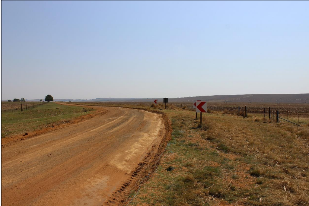
Figure 37: View north from Viewpoint MP3 – Pre-Construction
