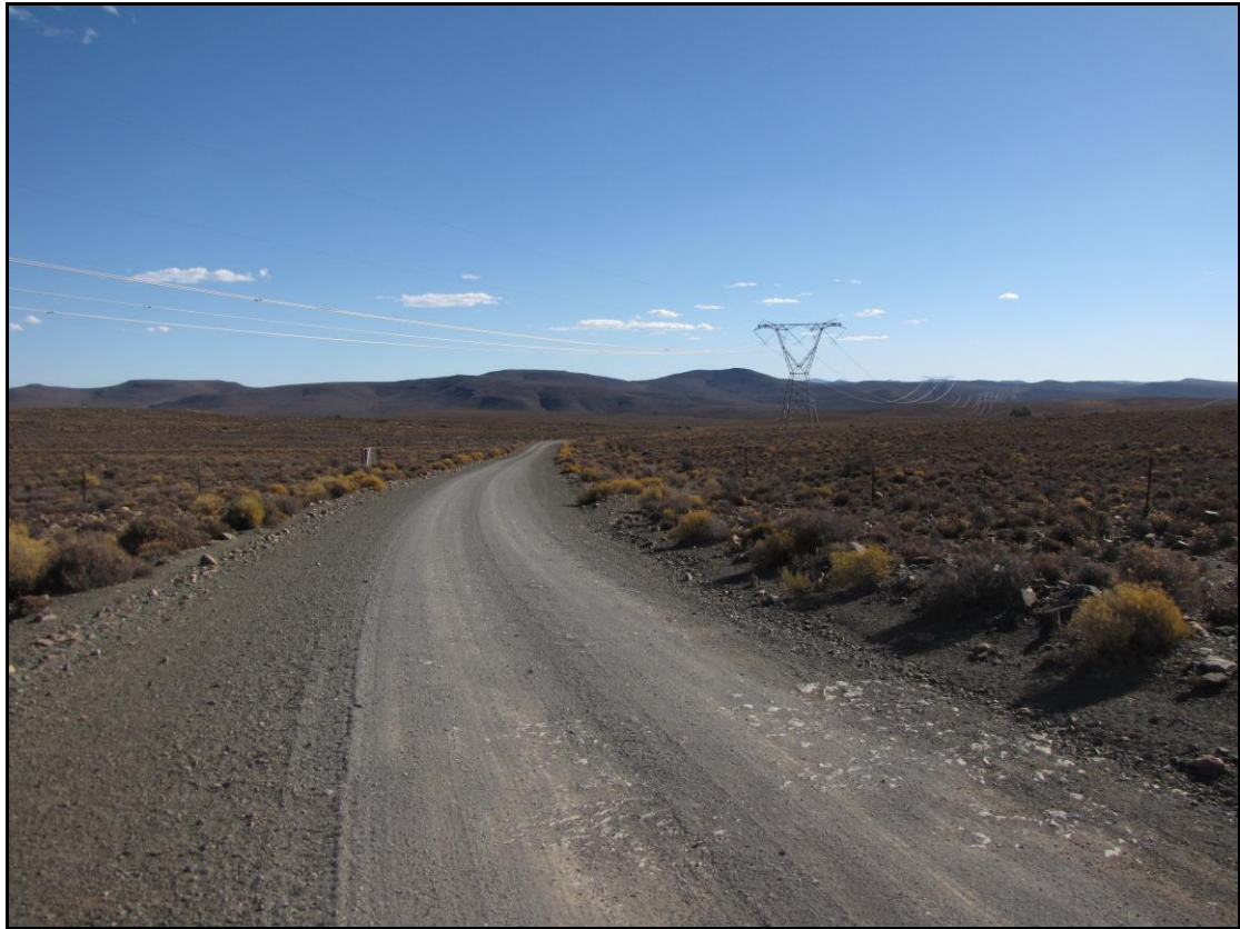
Figure 9: Existing power lines in the study area.
