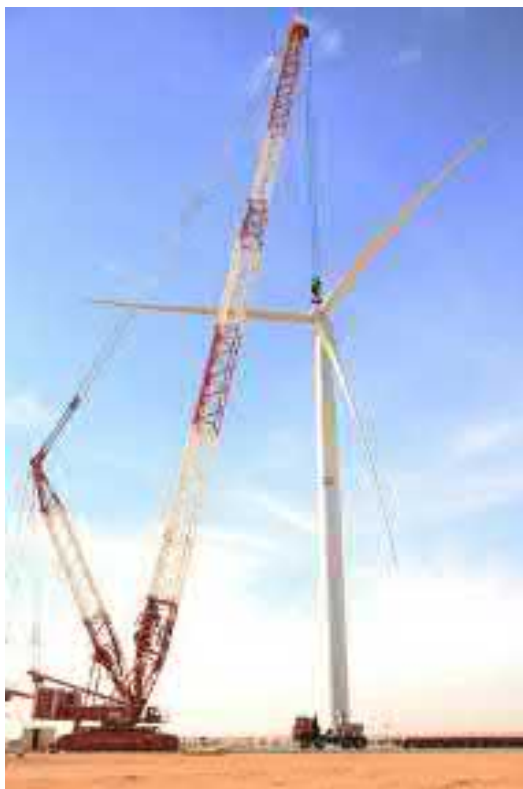
Figure 4-5: Crawler Crane used to assemble turbine (Liebherr, 2017)
