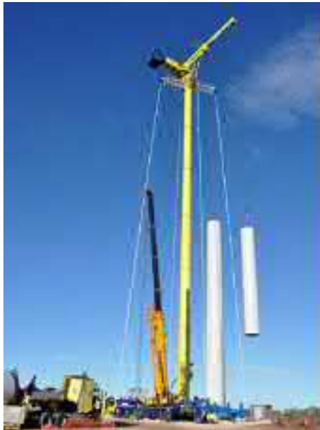
Figure 4-6: Cranes at work
