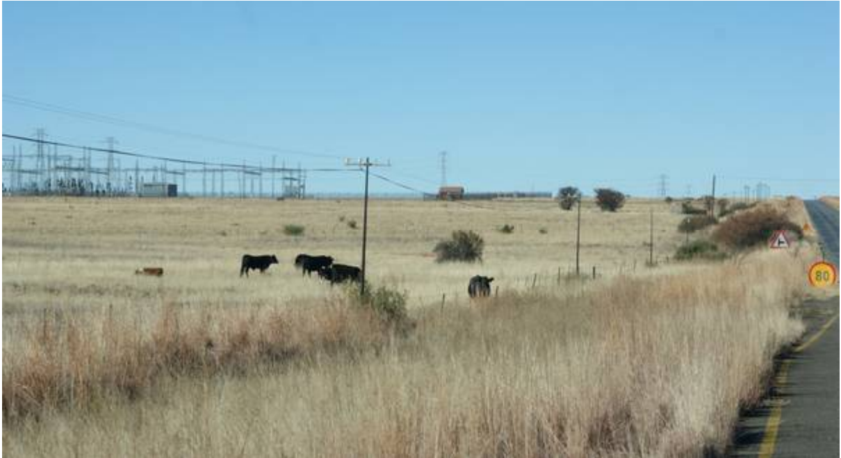
Photograph 3: View towards the project site from the R703 / 709 intersection.
