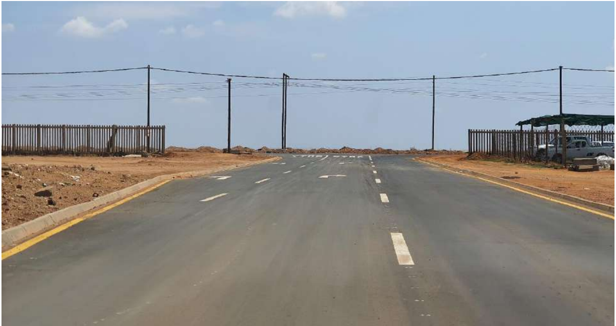
Photo 9: Looking west along Road D approaching the N11 (recently constructed new intersection adjacent the Site which on the right.
