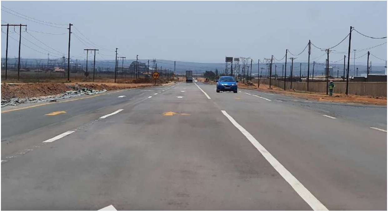
Photo 4: Looking north along the N11 near the new Road D intersection (Site is on the right behind the wall)
