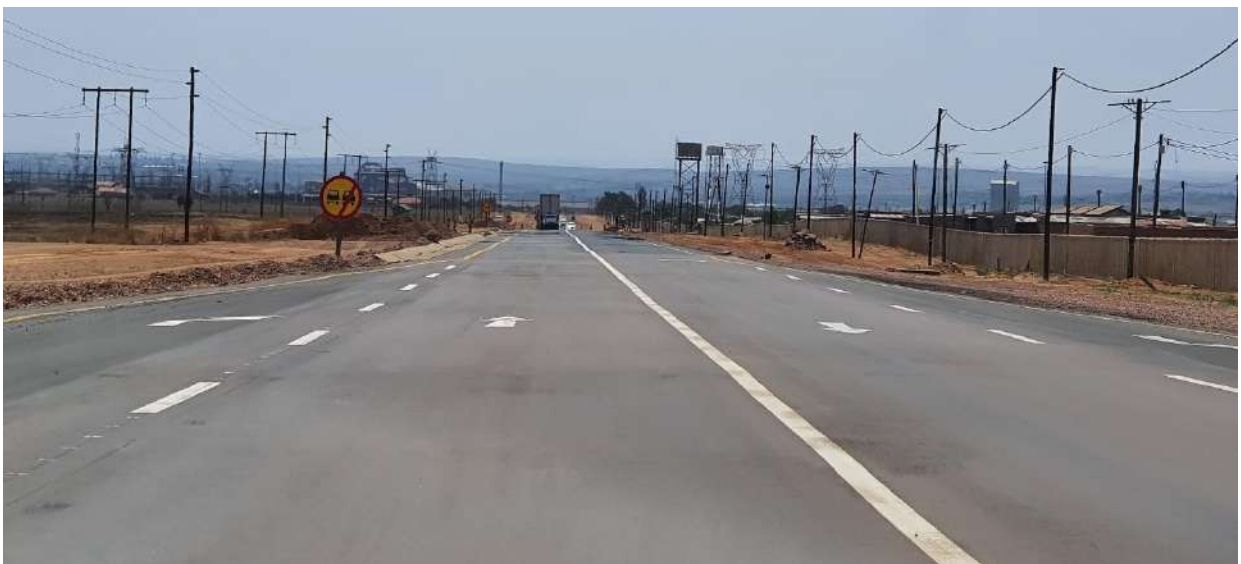
Photo 5: Looking north along the N11 leaving the new Road D intersection
