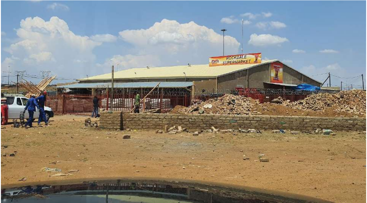
Photo 8: Looking south-east at the internal Rockdale Supermarket along Road D
