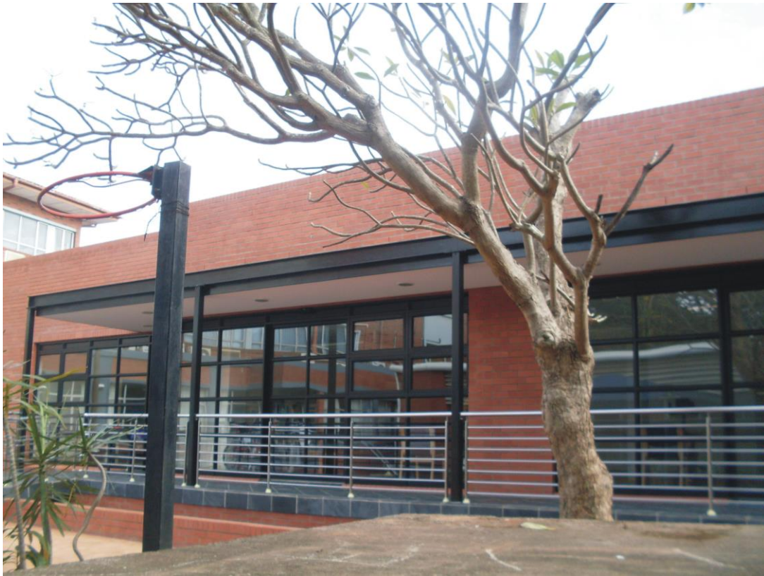
Photo 6: Existing modern rehab building
