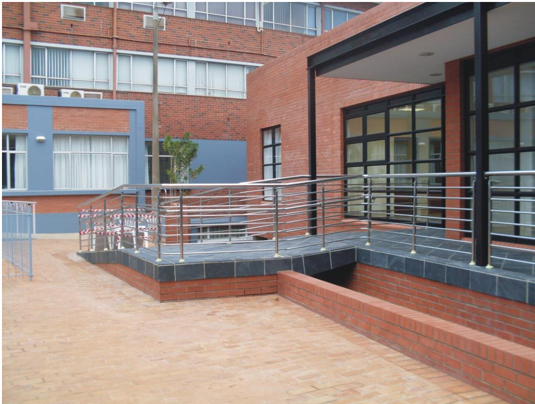
Photo 7: Existing modern rehab building
