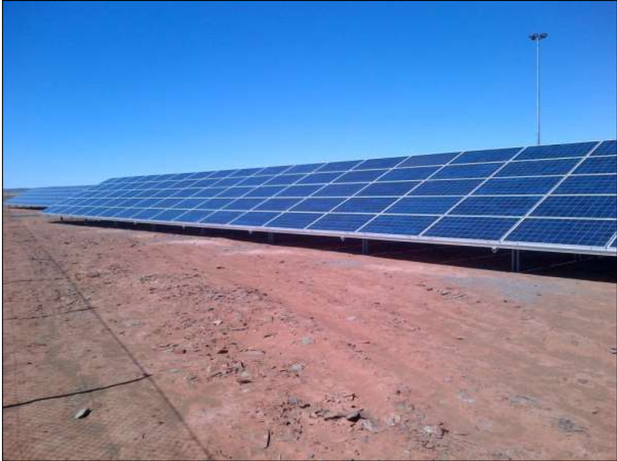
Figure 43: Photovoltaic Panels being erected near De Aar in the Northern Cape Province
