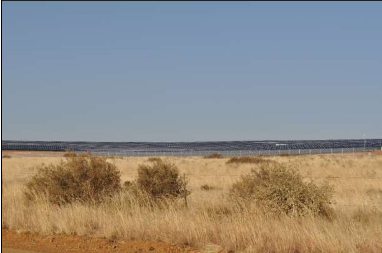
Figure 44: Photovoltaic Panels being erected near Lime Acres in the Northern Cape Province
