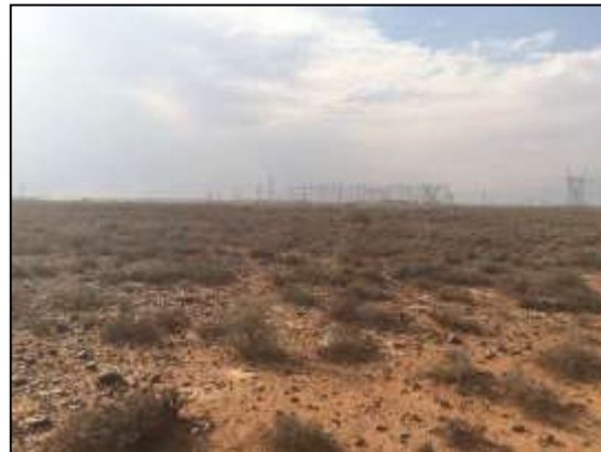
Figure 60 – View of northern corridor alignment with the Kronos substation in background
