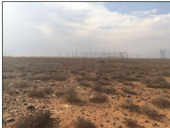
Figure 56 – View of northern corridor alignment with the Kronos substation in background
