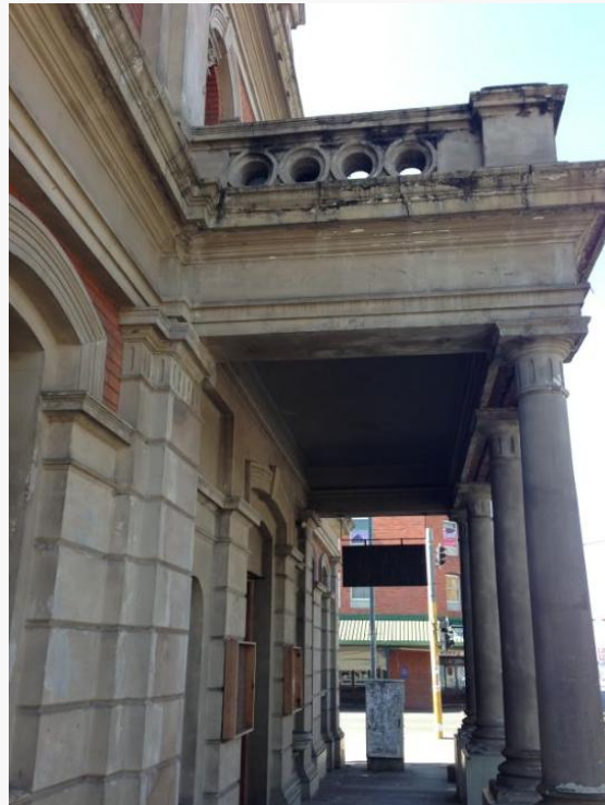
photo 16 above Flat roof over entrance portico shows significant staining, suggesting poor rainwater management
