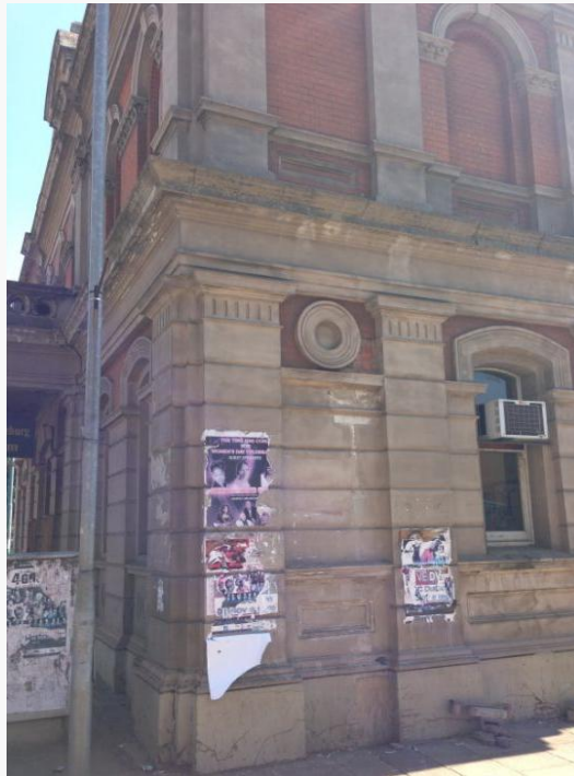
photos 5 & 6 Typical condition of plaster moulding – poorly maintained, significant cracking & frequently covered with layers of signage bills
