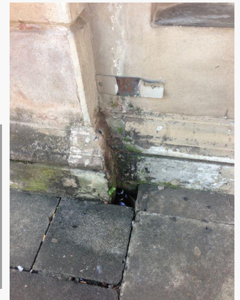
Photos 17 & 18 right Rainwater down pipe that should be serving the portico roof is missing, leading to damage to the surrounding render
