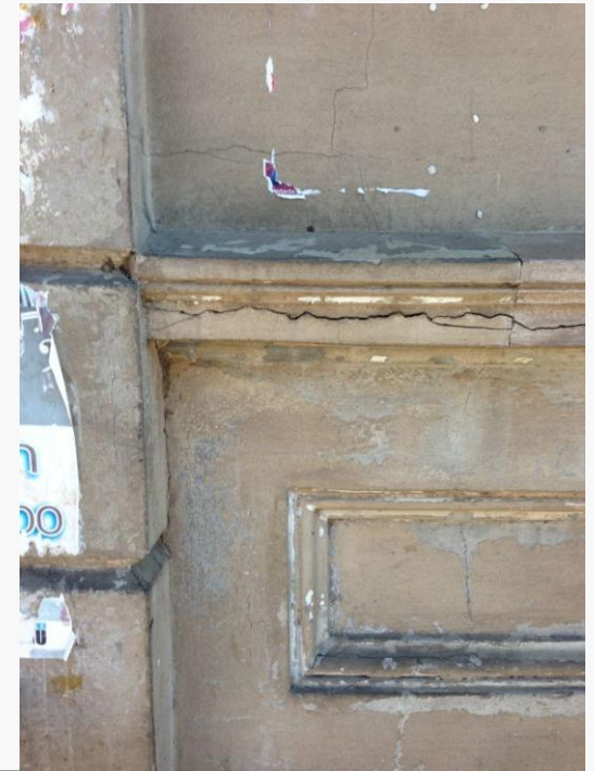
photos 5 & 6 Typical condition of plaster moulding – poorly maintained, significant cracking & frequently covered with layers of signage bills
