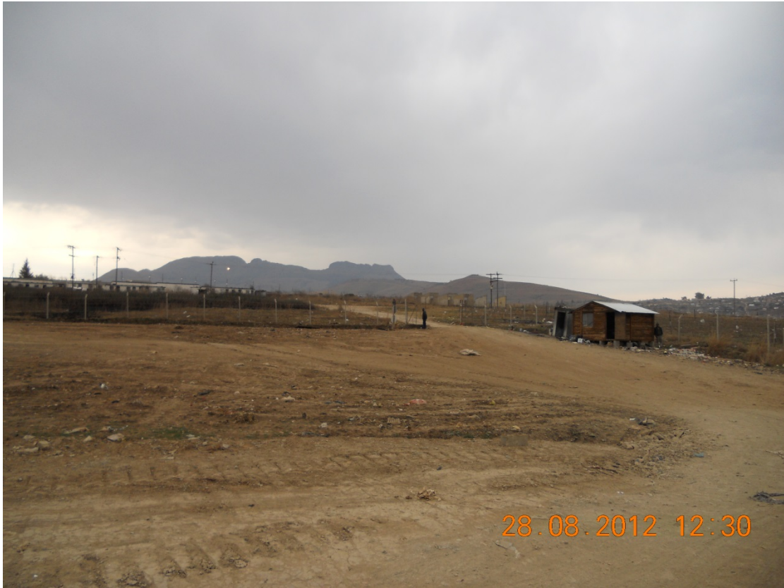
Figure 9: Site entrance with guard hut
