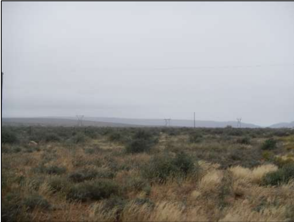
Figure 135: View of the existing high voltage power lines that can be found within close proximity to the proposed Aletta Wind Energy Facility application site
