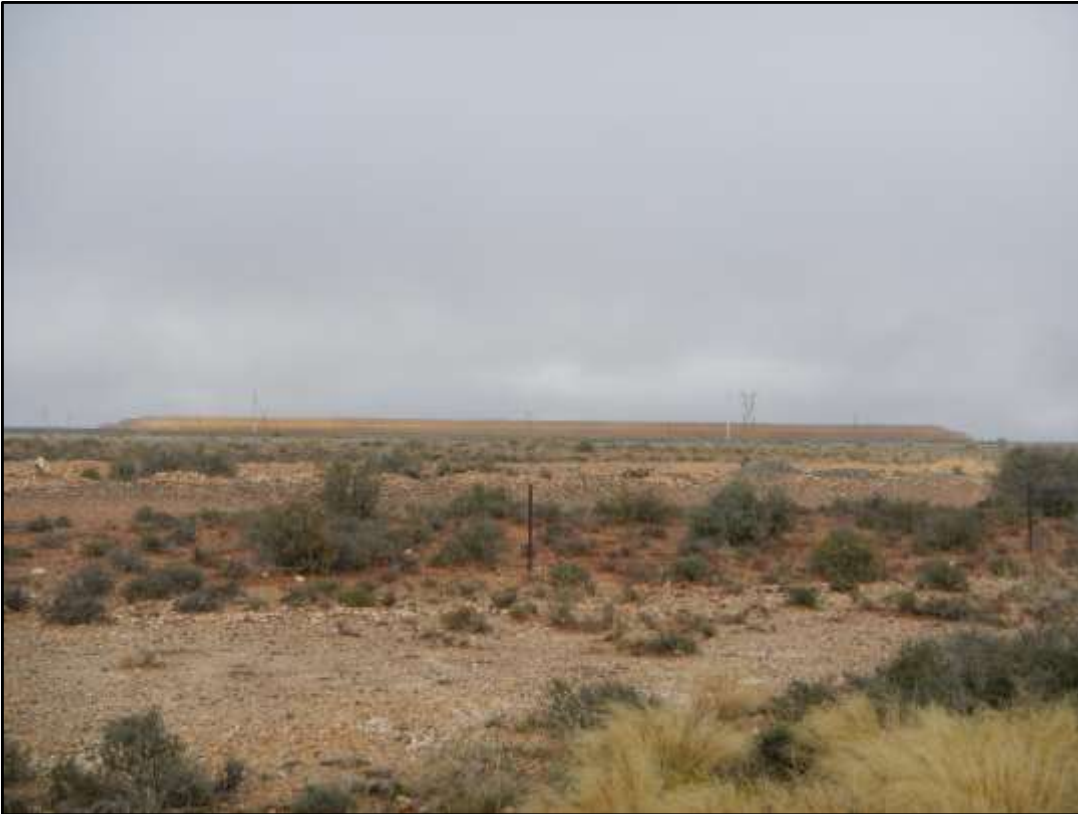
Figure 104: View of the Copperton Mine slimes dam which can be seen from sections of the R357 road. The south-western gravel section of the R357 road passes close to this slimes dam
