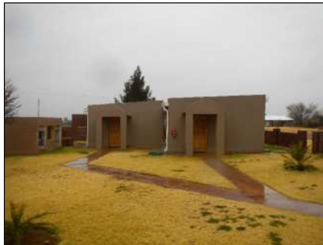
Figure 109: Typical views of the guesthouse buildings / facilities found at the Nelspoortjie Karoo Guest Farm (VR 2).
