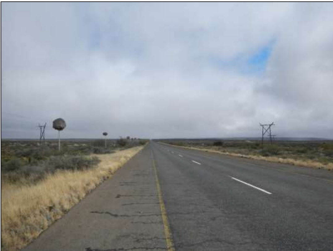
Figure 105: Photo of existing high voltage power lines which traverses a section of the R357 tar road
