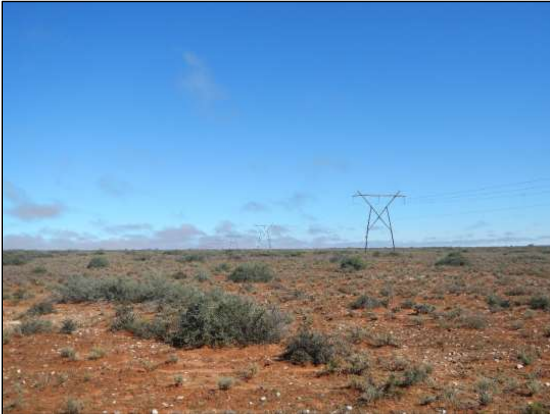
Figure 16: View of the existing high voltage power lines found within the surrounding area
