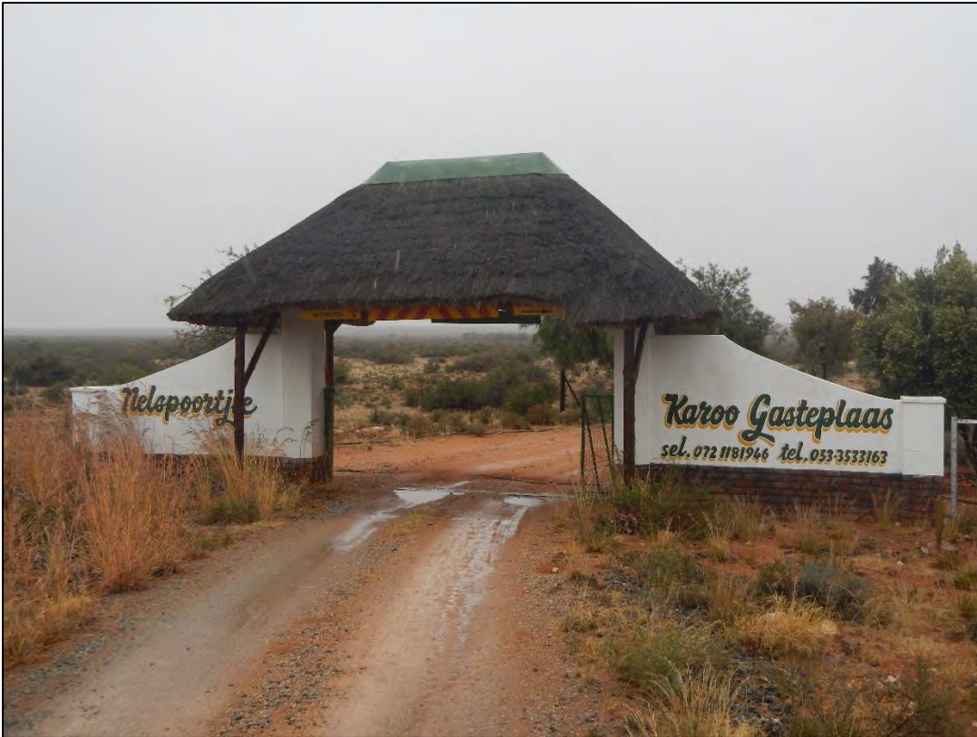
Figure 98: View of the entrance of the Nelspoortjie Karoo Guest Farm (VR 2) which is accessible via the R357 Copperton Road
