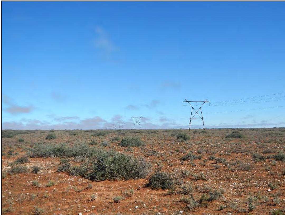
Figure 16: View of the existing high voltage power lines found within the surrounding area
