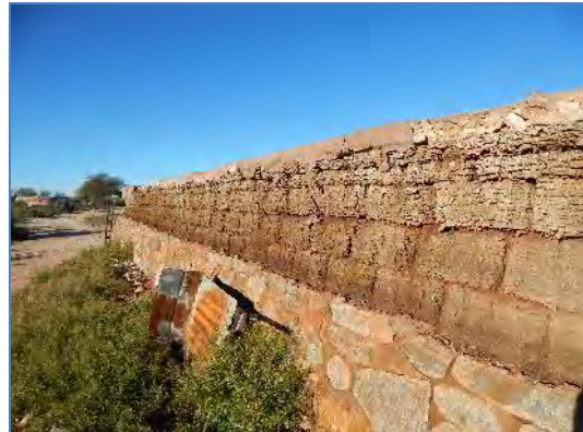
Figure 178: Exposed compressed dung bricks
