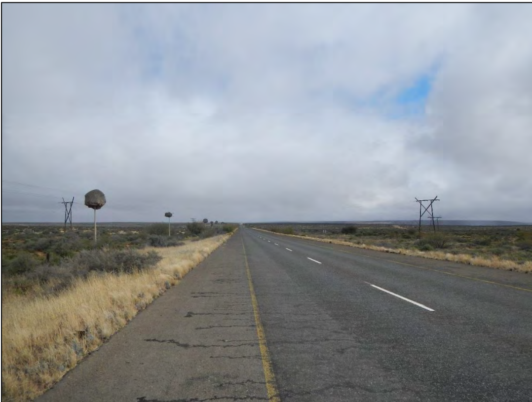
Figure 105: Photo of existing high voltage power lines which traverses a section of the R357 tar road
