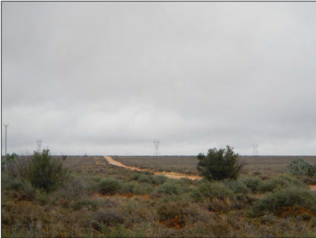
Figure 117: View of the existing high voltage power line which can be found to the south-west of the farmstead / residential dwelling at VR 11. This power line is expected to alter the natural / scenic character of the surrounding area slightly and lessen the visual contrast of the proposed Aletta Wind Energy Facility.
