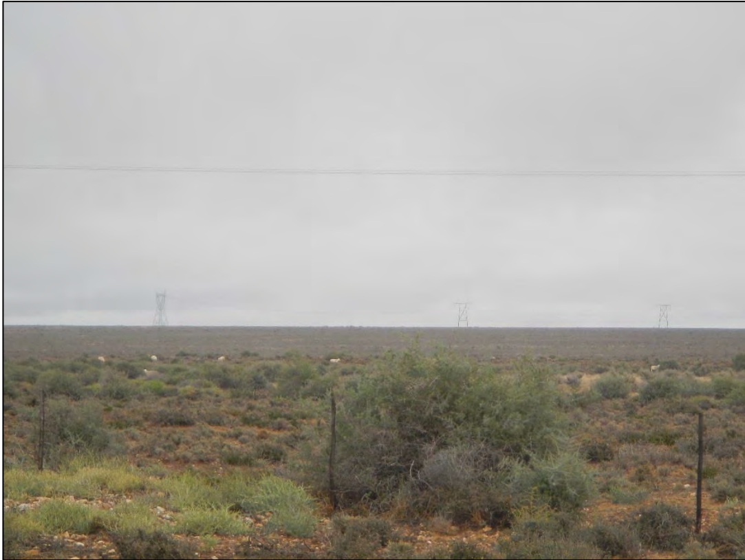
Figure 111: Typical view of the existing high voltage power lines that can be found to the south-west of the farmstead / residential dwelling at VR 4.
