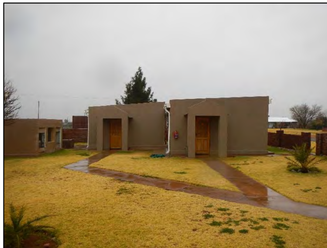
Figure 109: Typical views of the guesthouse buildings / facilities found at the Nelspoortjie Karoo Guest Farm (VR 2).
