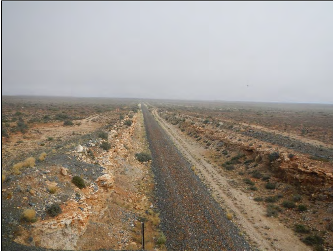
Figure 17: View of the non-operational railway line which traverses the northern section of the application site. Note that no railway tracks are present.
