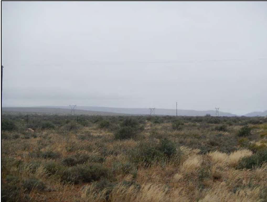
Figure 135: View of the existing high voltage power lines that can be found within close proximity to the proposed Aletta Wind Energy Facility application site
