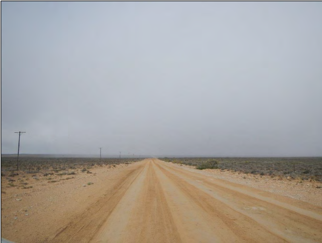
Figure 102: View of the south-western section of the R357 road which becomes a gravel road and provides access to the existing Kronos Substation
