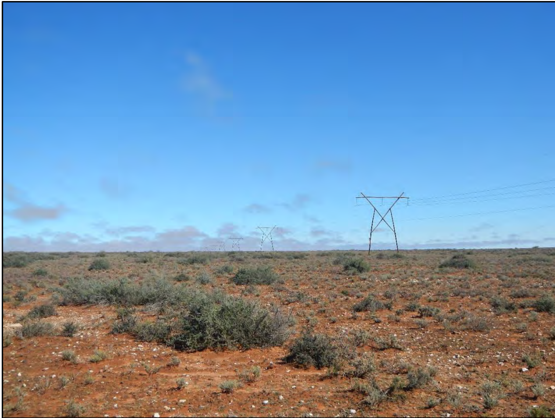
Figure 32: View of the existing high voltage power lines found within the study area which are expected to alter the overall natural / scenic character of the study area slightly and lower the visual contrast associated with the proposed wind energy facility.
